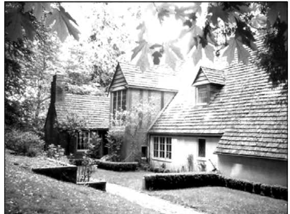
Noted architect Richard Sundeleaf designed and built this lakefront house in 1939-40 at Phantom Bluff in the English Cottage style for his personal residence.
