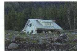
channelized debris flow
