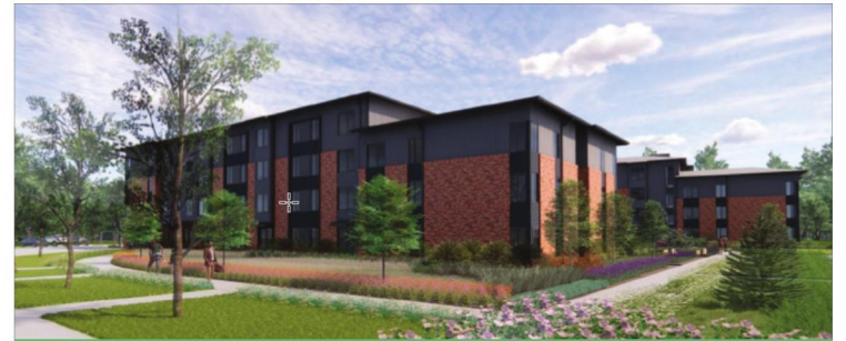
Mercy Greenbrae at Marylhurst Commons, a 100-unit affordable housing development completed in 2024
