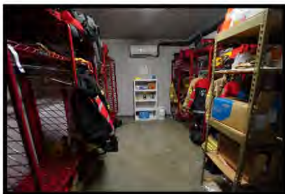
Figure 14. The existing turnout room is undersized.
